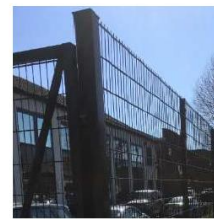
Existing fence and gate to be re-used
